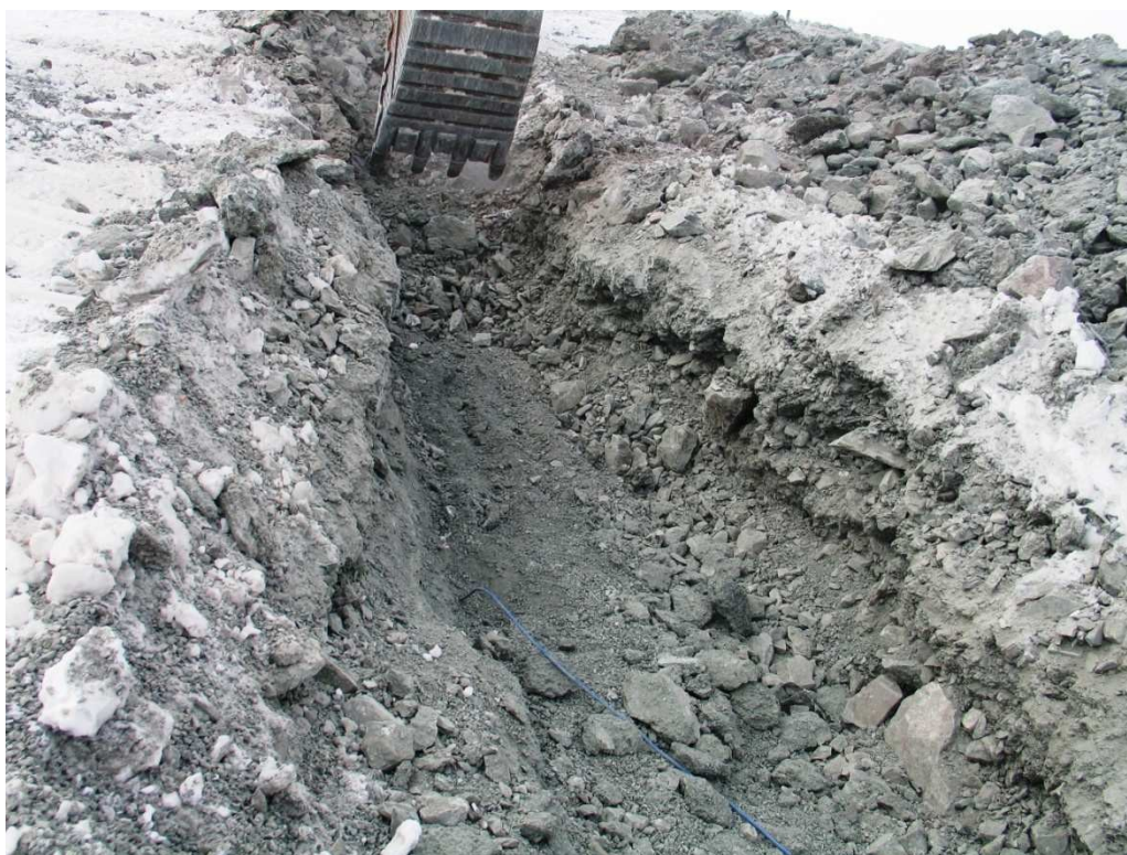
Photo 10: Cable exposed to ~ 1 m depth.
