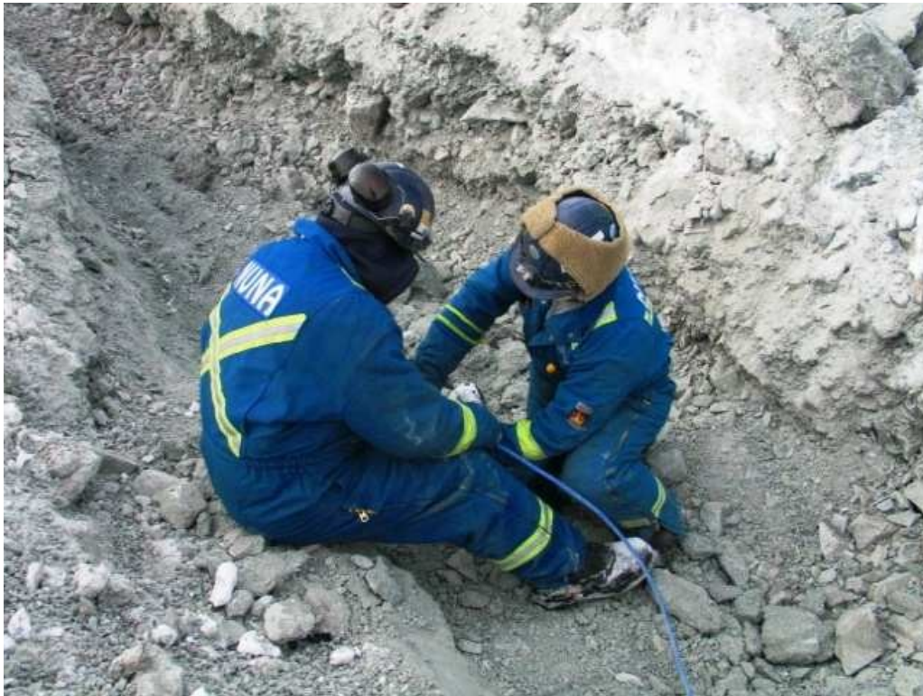
Photo 11: Electricians repairing nick in sheath of cable.
