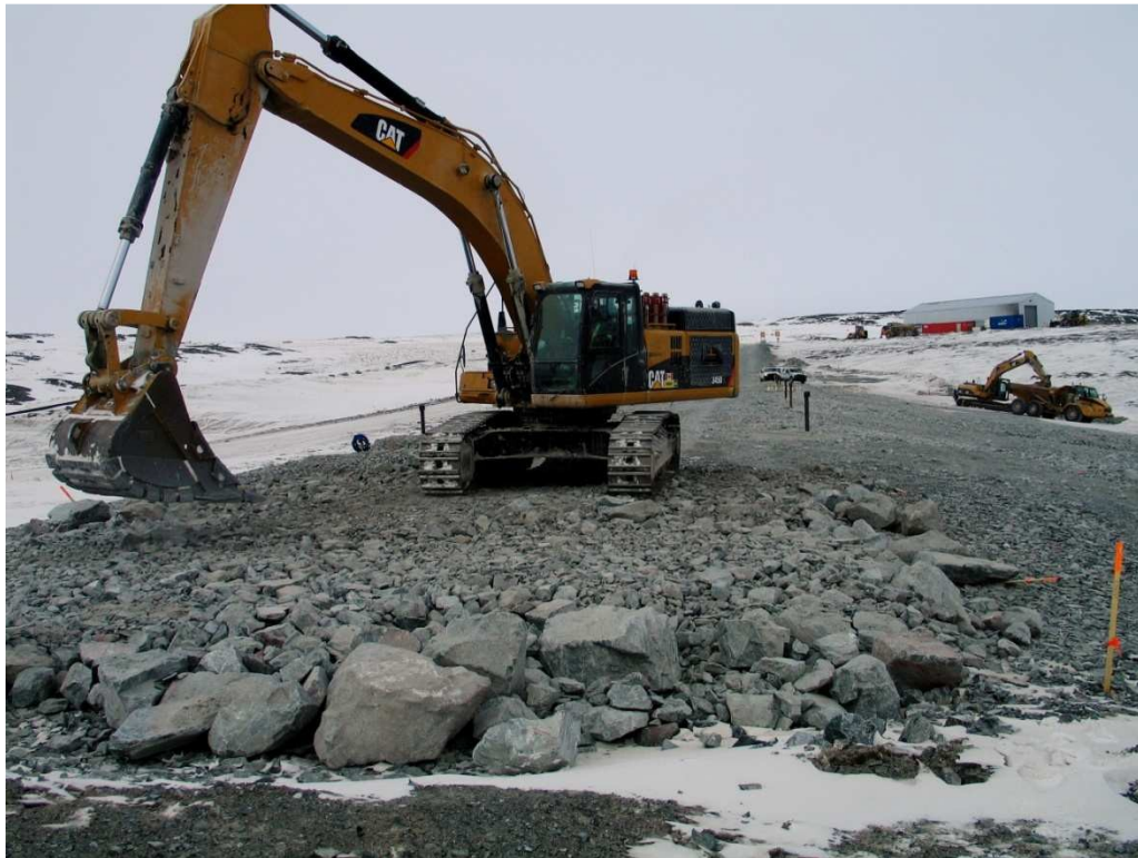
Photo 1: Excavator filling in low area at south end of dam.
