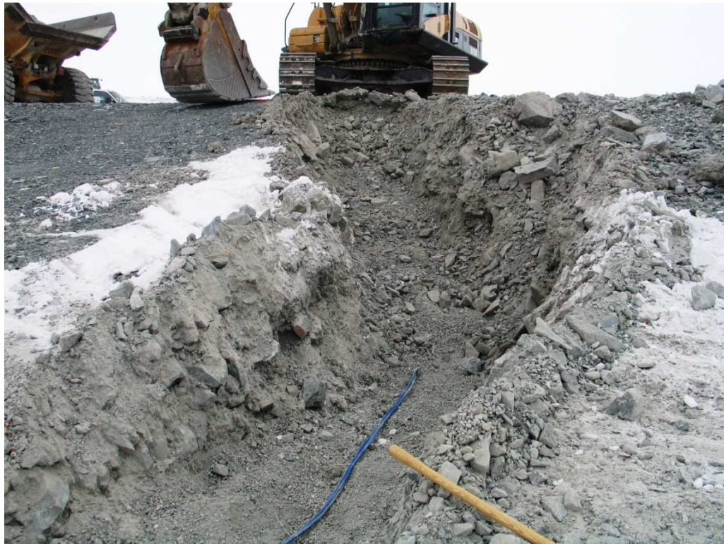
Photo 3: Cables that were placed at elev 33.5 exposed to a depth of 1 m. Sta 1+75. Curve to end at point shown on IFC drawings
