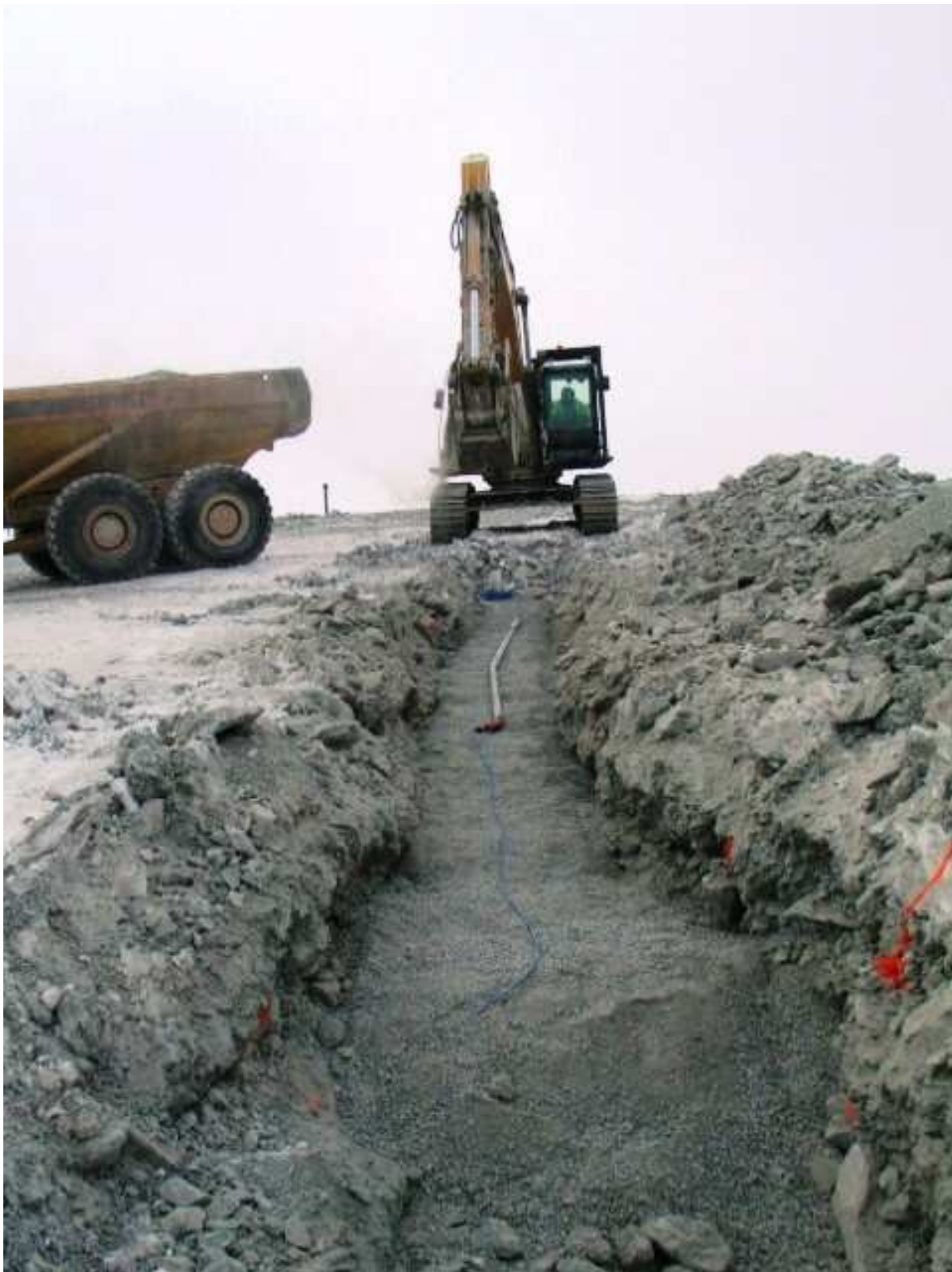
Photo 13: Progress for about ½ the shift. Cable is brought to center. Pipe will be buried as cable is frozen in the pipe. Operator reported that this trench was more difficult to excavate than the others.
