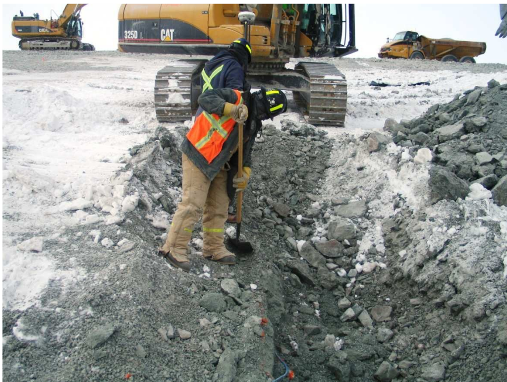
Photo 9: Trench excavated along side cable. Cable then chipped out
